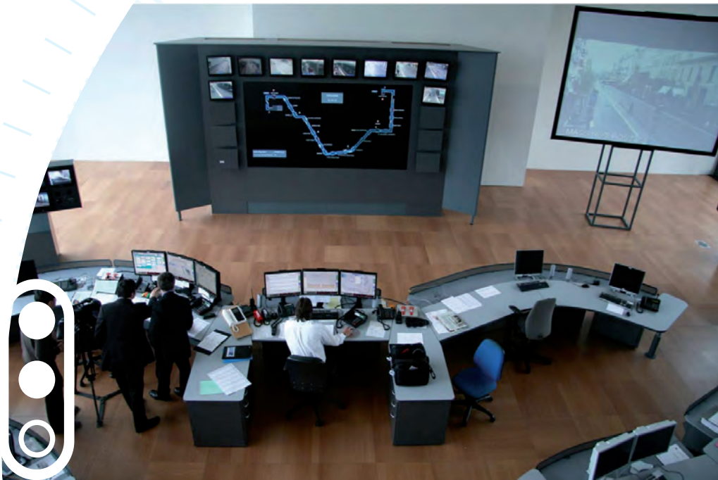
Panorama at the Nice Tramway Control Center.
