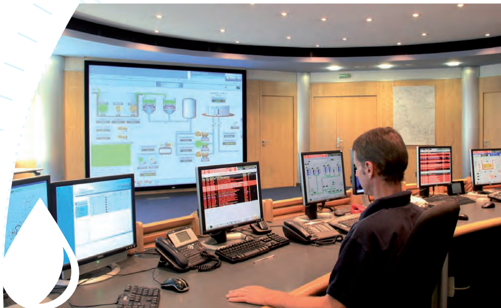
Panorama at the Telemetry Center of the Société des Eaux de Marseille. Permanent remote overseeing of over 850 hydraulic plants, real-time collection and treatment of almost 95,000 data points.
