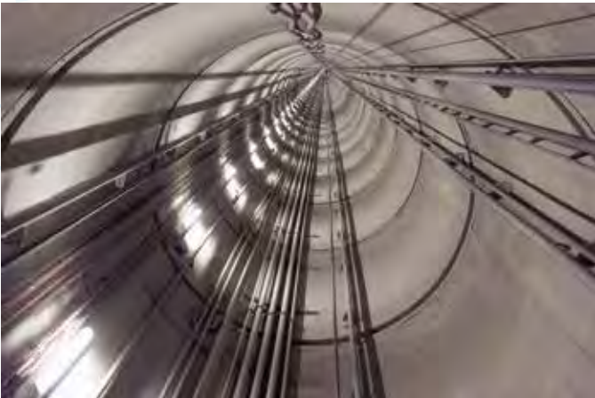
Well of access to the Andra underground Research laboratory - 490 m of depth.
