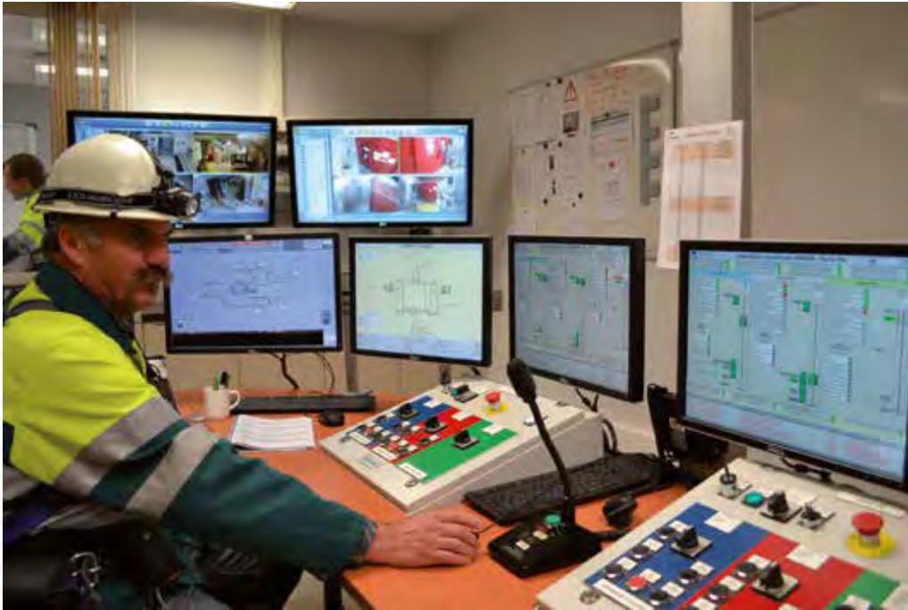
CCS : Andra Control-Command Station using Panorama SCADA software.
