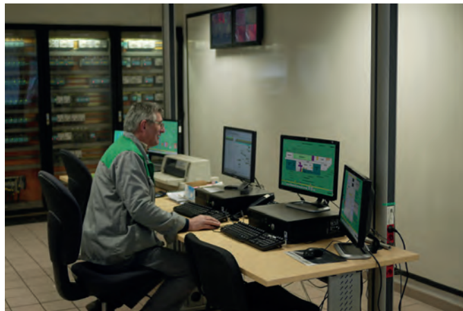
New remote control room
