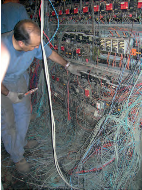
Dismantling of the LV room
