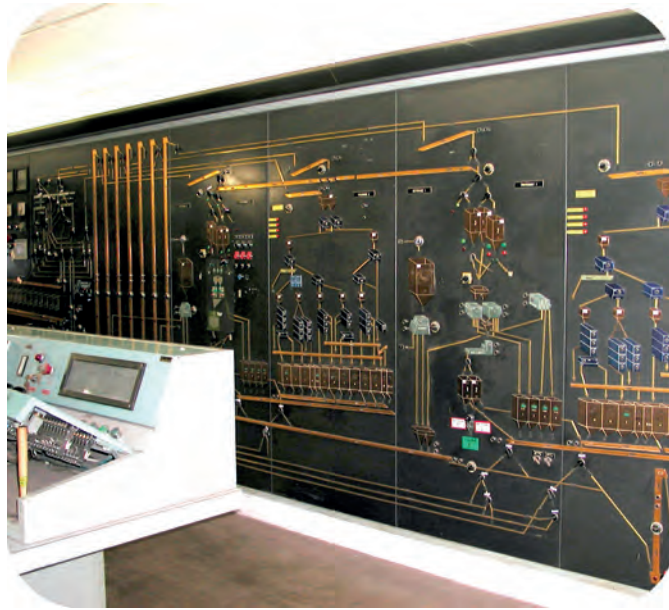
Former manual control room
