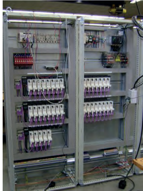
Renovated LV room
