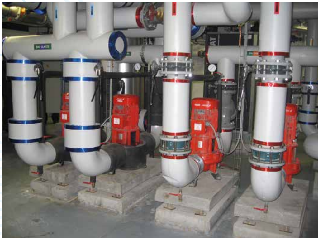
Equipments room containing heat pumps and condensers
