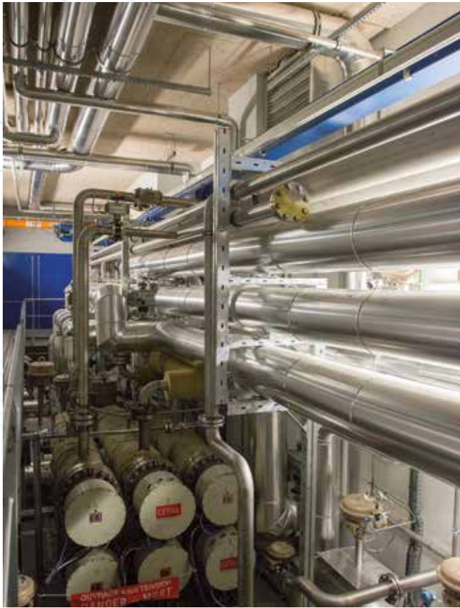
Compressed air distribution area used to deliver air to the test rigs as required.
