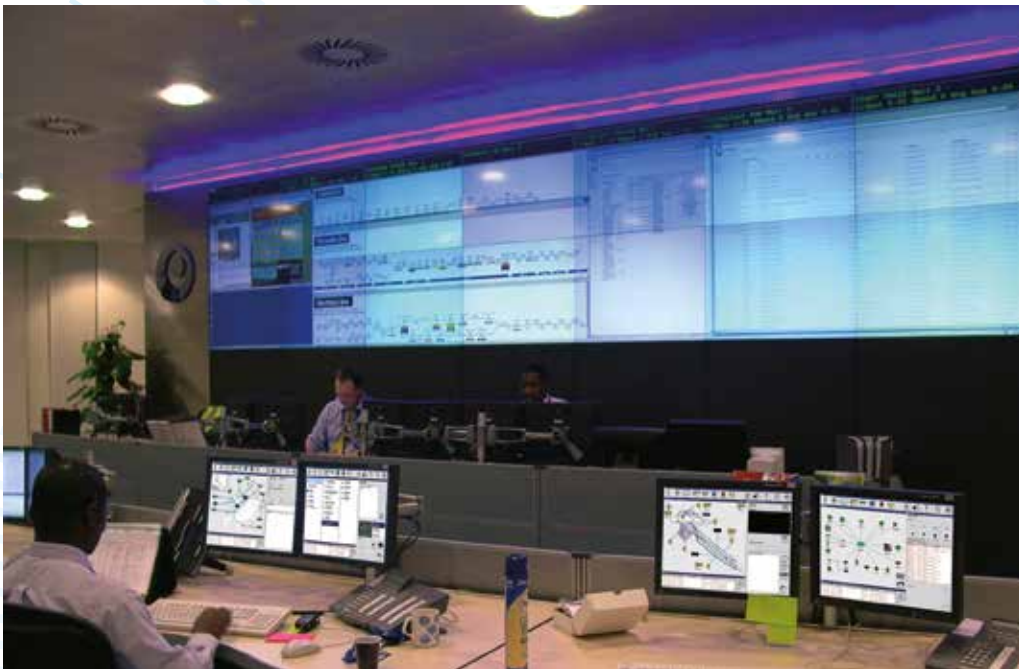
Panorama E 2 used at Tube Lines control center
