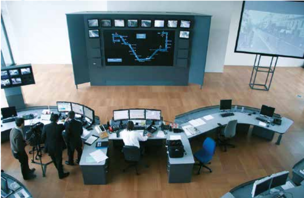
CCC: Central Command Centre in front of the operators is the OCP (Optical Control Panel) managed by Panorama E 2 , which provides information on the status of the tramway line.
