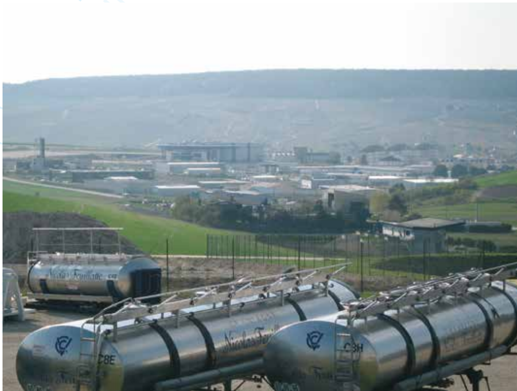
Collect must & water purification plant
