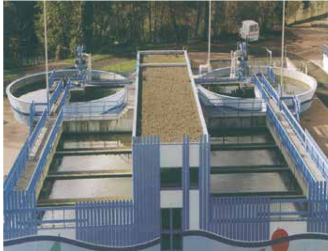
Drinking water plant located at Gour du Puy, Montluçon - France
