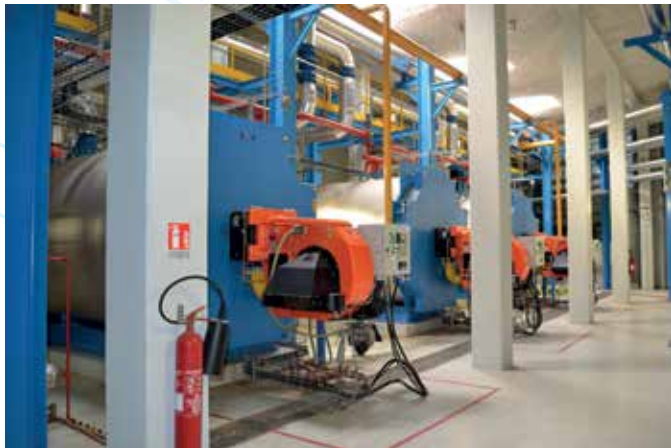
Heating capacity of 24 MW produced by 3 hot-water boilers
