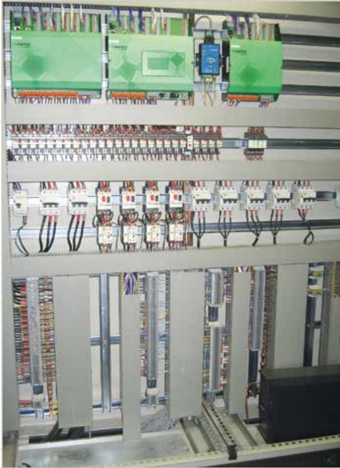
Controller cabinet : Linking Sauter controllers to other plant equipment
