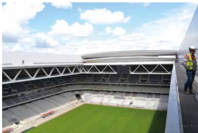
The first French stadium with a retractable roof, comprising two 7,200 ton rigid sections, that open in just 30 minutes.
