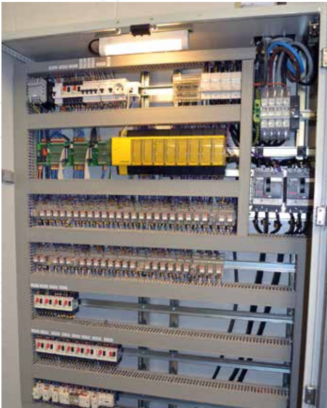
Wiring closet : Linking the controllers to all the technical equipment.
