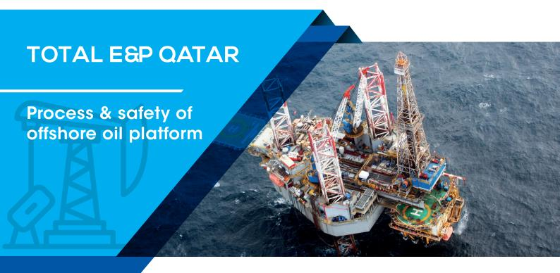
Total Exploration & Production Qatar (TEPQ) operates the Al Khalij oil field, located 130km off the coast of Qatar. The process of oil extraction involves several stages: first, the oil is extracted by a cluster of 7 unmanned platforms and piped to the island of Halul 40 km away. There, it is processed by two separation trains and stored before being transferred to oil tankers towards the refinery.
